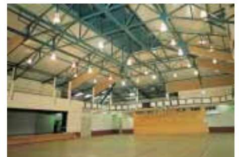
Above: Sandwich panel roofing at the Cooloola Sports Centre. Top left: Sandwich panel wall system at Arnott's facility, Sydney.
