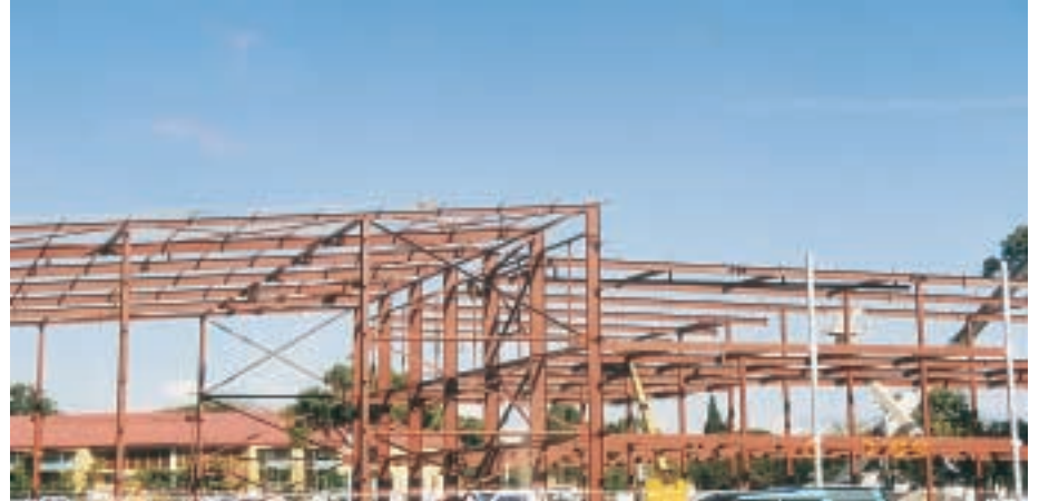
Above: Construction of unprotected steel frame in July, 1999.
